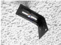
Using either the included wood screw or the included toggle bolt, attach the L-bracket to the ceiling. (Note: Some of the toggle bolts shipped in May were a bit oversized. You may need to use a different toggle bolt. "No good deed...").;)
